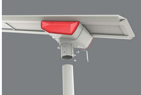
(2). Fasten the 6 screws with tools
